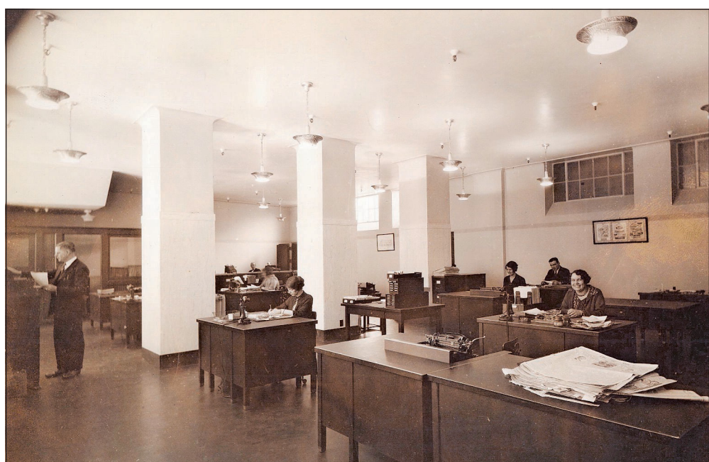
THE DAY The first-floor business office in 1929, after the expansion of the building was completed.
